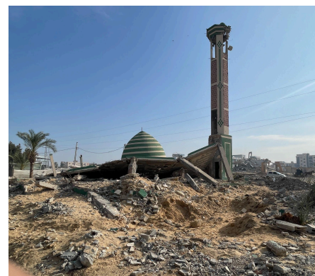
UNMAS EOD Officer conducts an EHA of a damaged mosque as part of UNDP Debris Management efforts. Deir al Balah, Gaza, 6 January 2025.
