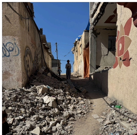
EHA as part of UNDP Debris Management Pilot Project, conducted on 26 October 2024 in Dair Al Balah
