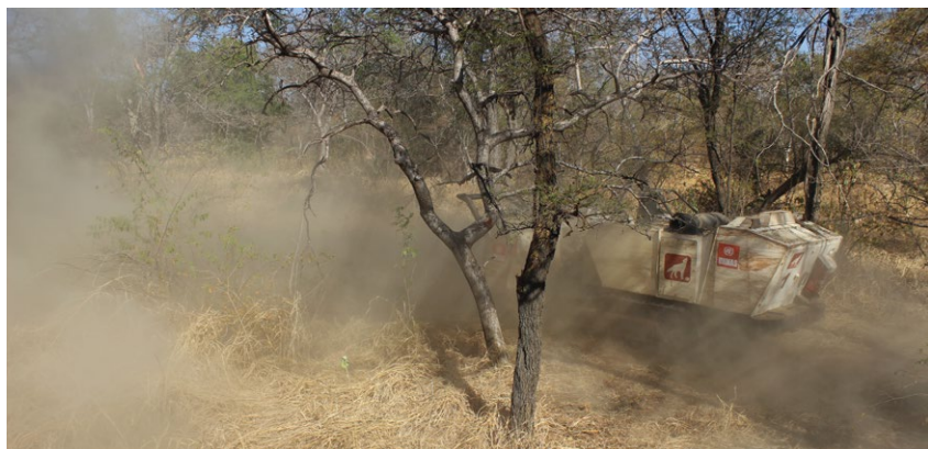
Minewolf mechanical vegetation clearance at TS 12 As Sumayah/War Abar
