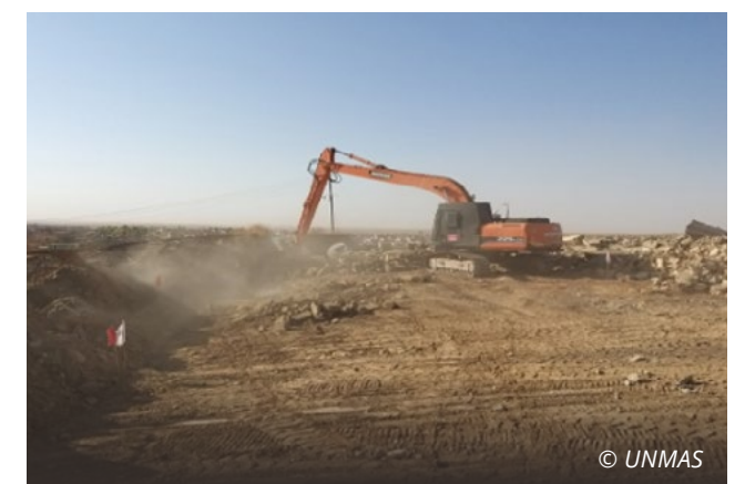
UNMAS implementing partner (G4S) using armored excavator in removing rubble from the police compound in Sinjar.
