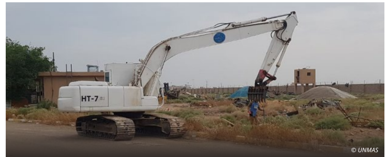
Mechanical clearance utilising raking with the excavator.
